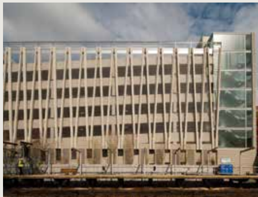
Photos courtesy of Unistress Corporation, Pittsfield, MA.
